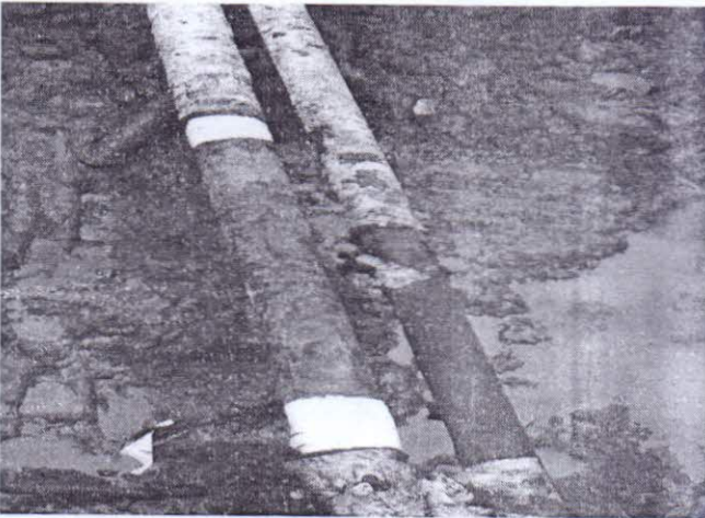
FIGURE: 3 REPAIR WORK
